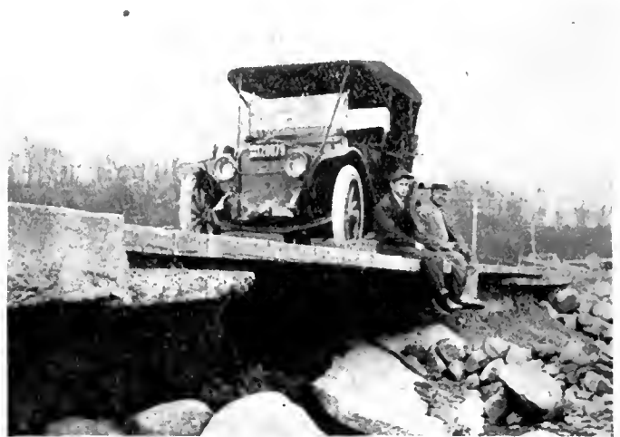
A severe test on the strength of lateral bonds in grouted brick pavement.
